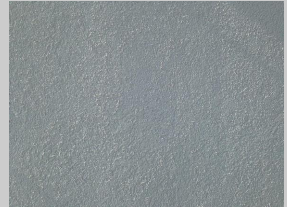
after being coated with KaWaTech
